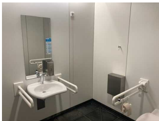
Public toilet, men
